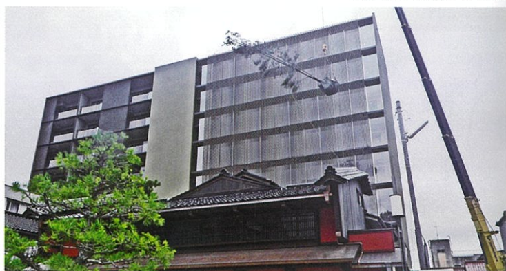
アカマツ搬入 施工中 During Construction: Bringing the Pine Tree ( ' 15.09)
